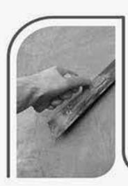
The surface where the tiles are to be laid must be properly finished and should not be uneven.
