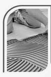
Neat cement should not be used for fixing tiles. Doing so may lead to cracks on the surface of the tiles due to hydration heat generated by cement. Tiles should be fixed either by cement & sand mortar as per the suggested ratio by engineer or architect or a good quality tile adhesive.
