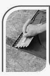
Before fixing the tiles, dry layout of tiles should be made in the desired pattern to ensure an acceptable blend of shade and design. Then fix the tiles with cement mortar or adhesive. Please note that certain amount of shade and size variation is inherent in the manufacturing of tiles. The company will bear no liability after the tiles are fixed.
