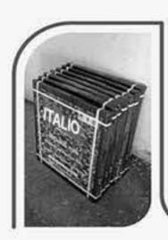
After receiving the tiles at site, first please segregate the tiles boxes according to batch no. & manufacturing date. Before laying, tiles boxes should be stacked vertically to avoid breakage & chipping in tiles.
