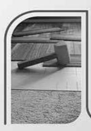
For proper bonding, press the tiles gently with a wooden mallet to make proper adherence. DO NOT USE AN IRON HAMMER OR SOME HEAVY MATERIAL TO PRESS THE TILE.
